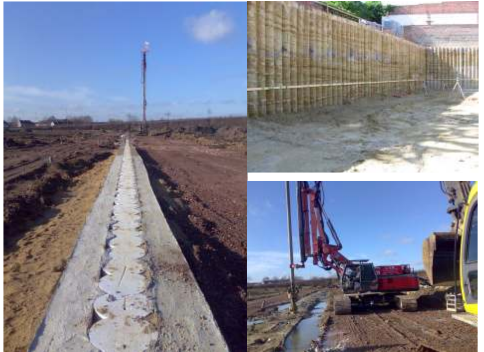
Secant wall made with grout through drill system
